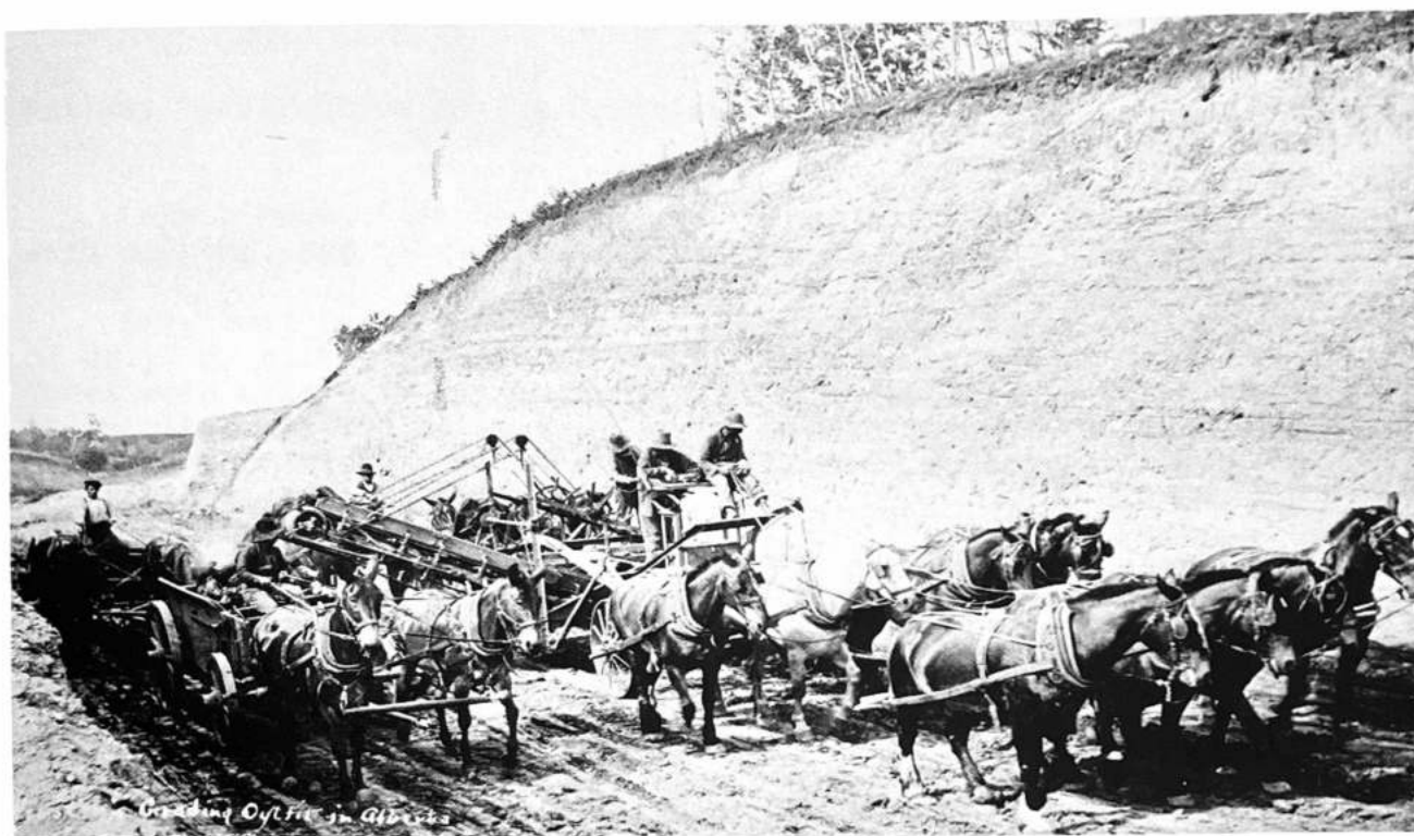
Photos 8 & 9. Cuts were excavated with elevating graders; earth being ploughed and loaded into dump wagons for haul and building up embankments.
