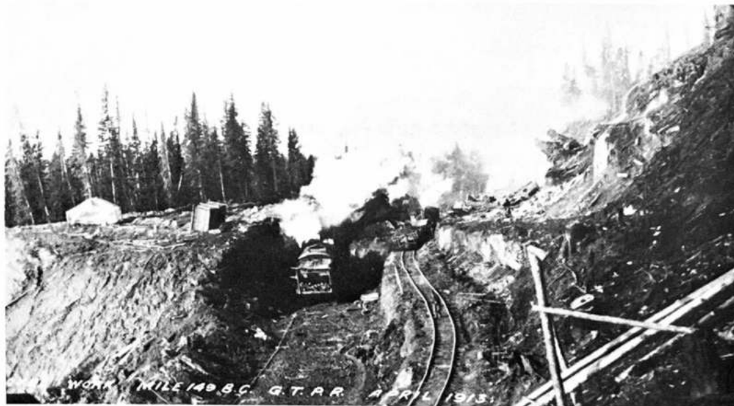
Photos 31 and 32. Construction of G.T.P.R. in the Upper Fraser Valley, heavy excavations were made by steam shovels and material was hauled, by dinky steam locomotives; to be dumped from high temporary trestles to build embankments.
