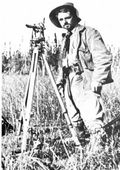
Photo 44. Knee-deep in muskeg with transit on pegs for some stability.
