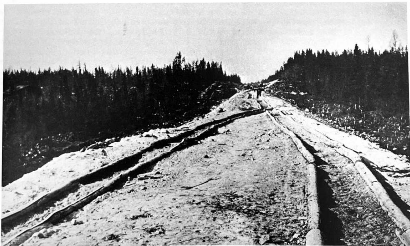
Photos 52 & 53. Excavating a cut, of glacial till, and loading it into cars, made on the spot, to be hauled over rails of local poles to build the adjacent embankment entirely by hand, near present time Gillam. Note, the double flanged car wheels to run on the pole track, also the well-trimmed slopes, 1915.
