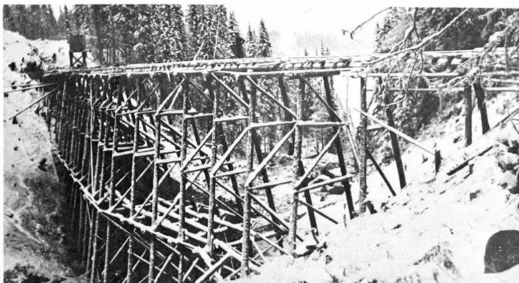
Photos 31 and 32. Construction of G.T.P.R. in the Upper Fraser Valley, heavy excavations were made by steam shovels and material was hauled, by dinky steam locomotives; to be dumped from high temporary trestles to build embankments.
