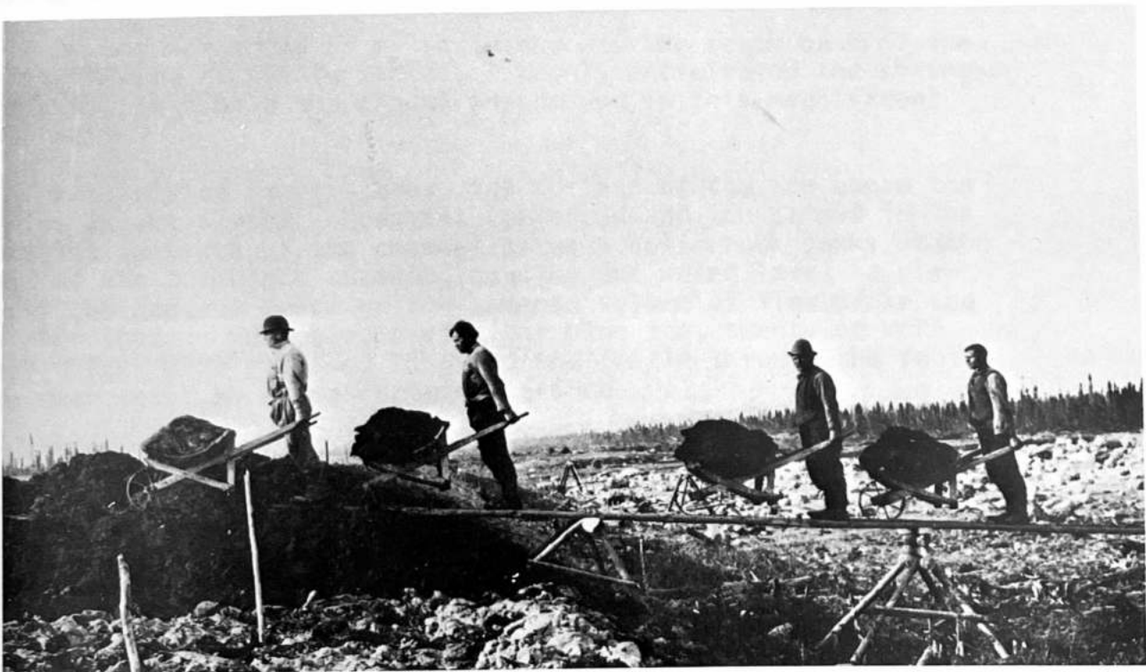
Photo 51. "Stationmen" grading embankment, from side borrow, on the south approach to the bridge site to cross the Nelson River at Kettle Rapids.
