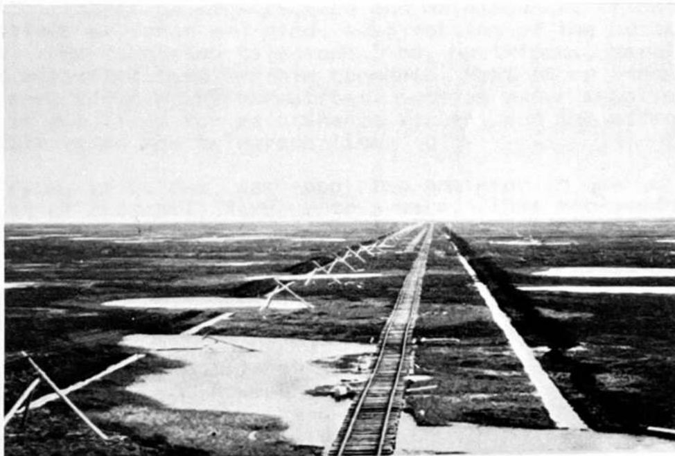
Photo 82. Skeleton track was laid into Churchill, 29 March 1929; this shows it across the "Barrens" at spring break-up when train-filling and hacking was commenced to build embankment and subsequently ballast the new railway. Note telegraph line on tripods.
